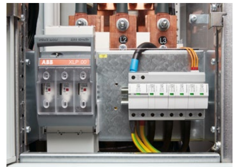
Surge protective device capable of carrying lightning currents
